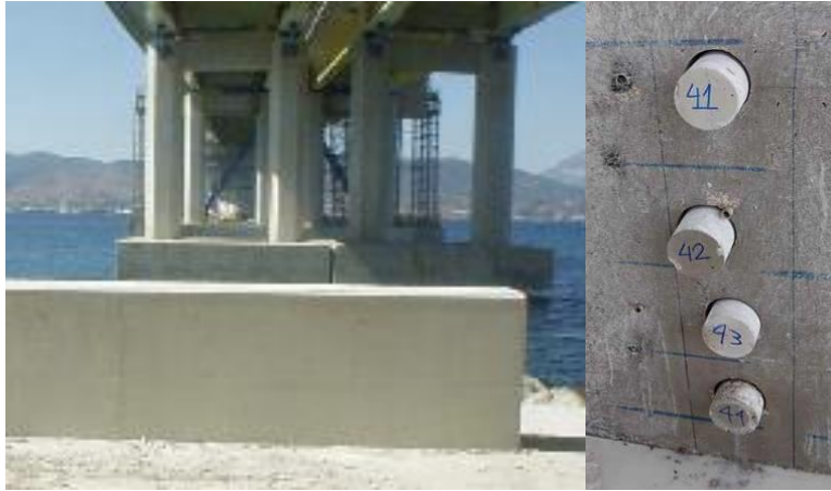
Sacrificial concrete block at P2 of Rion Approach Viaduct for concrete durability monitoring
